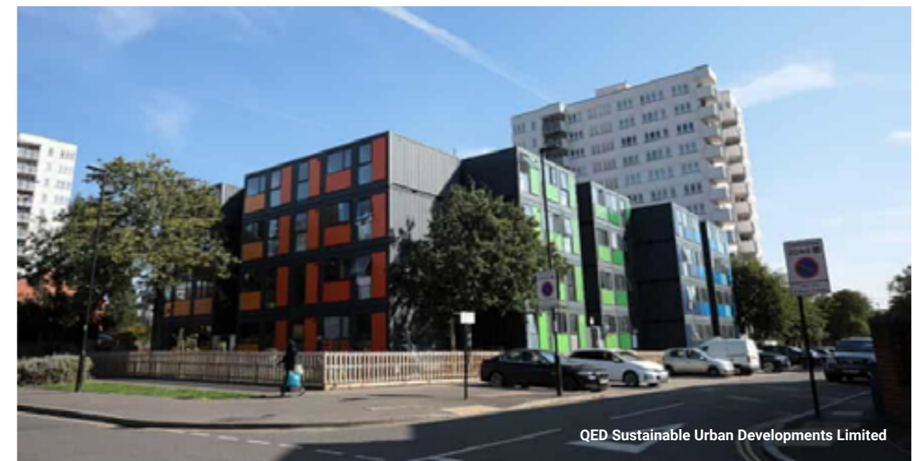
Figure 8 Shipping container flats at Meath Court, Acton
